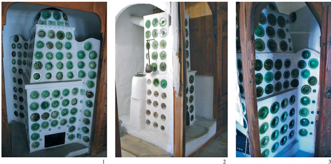
Fig. 31. Stoves in the Svrzo House in Sarajevo (Bosnia and Herzegovina), 18th century. 2. Next to one stove is a small steam bath ( hamamjik ) (Photographs: ©Gyöngyi Kovács)
